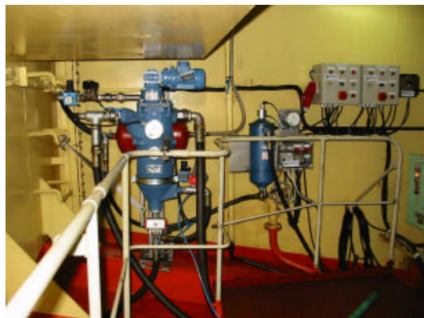
Picture 2: test plant M& RSK ARUN
